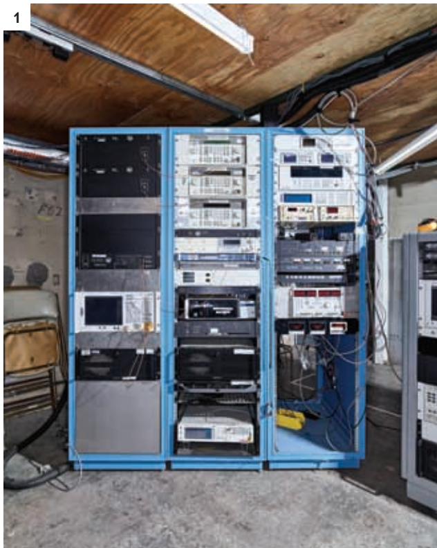
EQUIPMENT RACKS house ADMX's room-temperature microwave electronics (1). Engineers study sensor data from the experiment (2).
